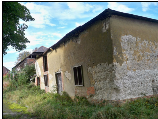
Cob barn to be demolished
